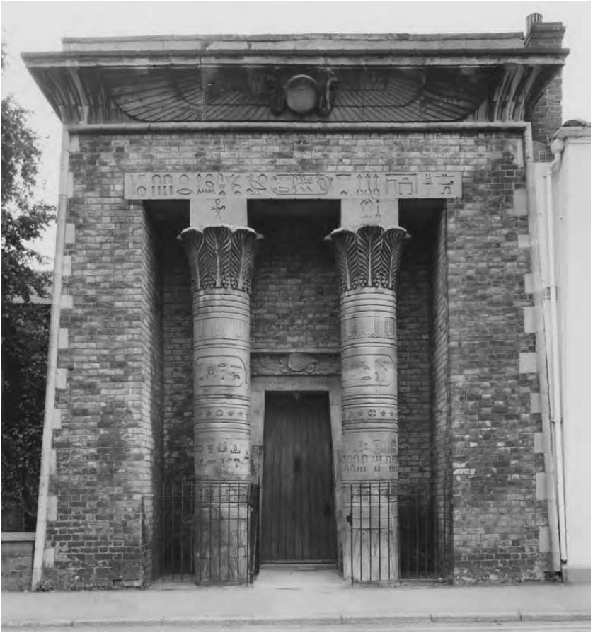
Plate 192 The Freemasons' Hall, Mainridge, Boston, Lincolnshire, of 1860–63. A powerful and archaeologically correct evocation of an in antis arrangement of portico in the Egyptian style constructed of yellow brick with limestone dressings. The inscription on the lintel above the palm-capitals reads 'In the Twenty-Third year of the Reign of Her Majesty the Royal Daughter Victoria, Lady Most Gracious, this Building was Erected' (Addys [Boston] Ltd, No. 12168A, collection JSC).
